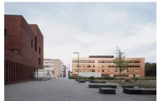
The Copper Coil - E-Technology Centre of the University of Rostock
